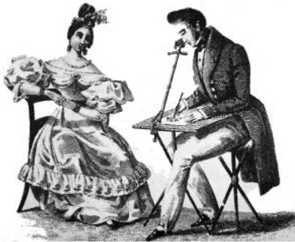
1807 engraving of a camera lucida in use.
